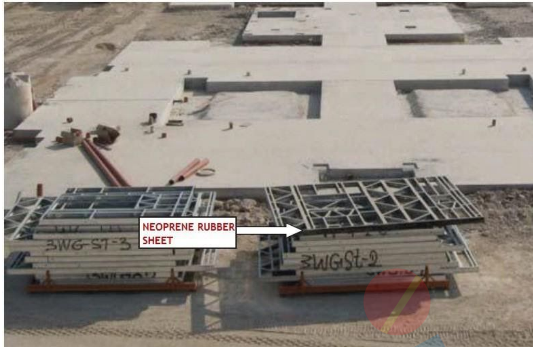
Fig 23. Neoprene Rubber Sheet at bottom of Wall Frame
