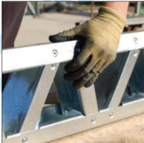
Fig 18. Typical Joist Assembly
